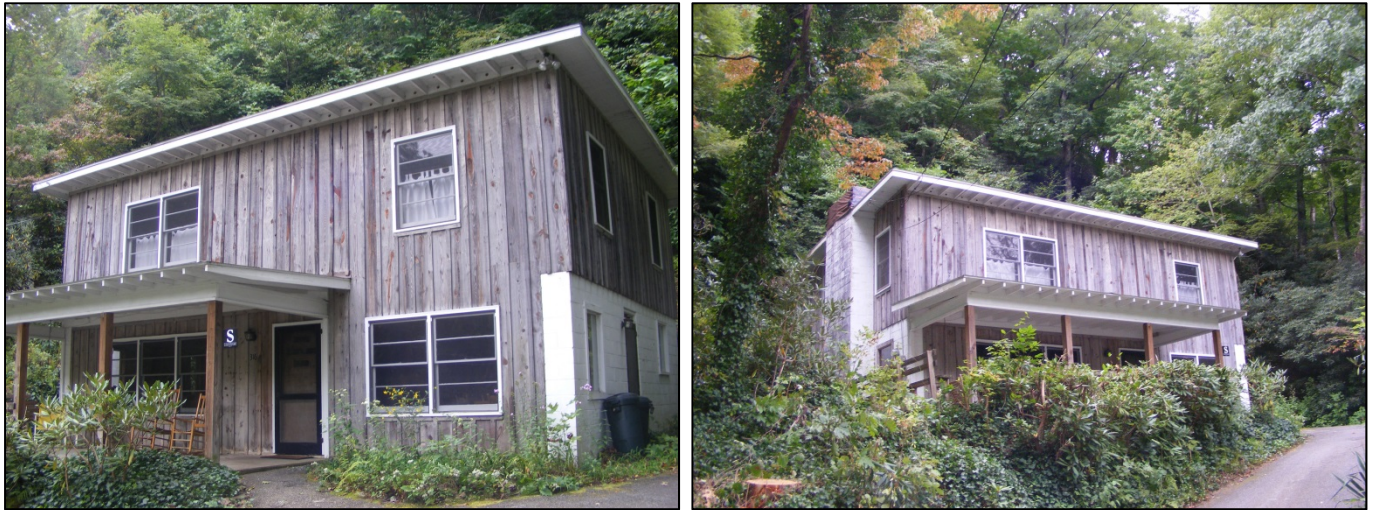
Figure 17. BN 5968: 316 Texas Road (Left; Façade and West Elevation; Right: Façade and East Elevation). TRC 2013.
