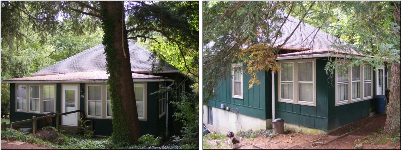
Figure 27. BN 5978: 224 Tennessee Road (Left: Façade and West Elevation; Right: Façade and East Elevation). TRC 2013.
