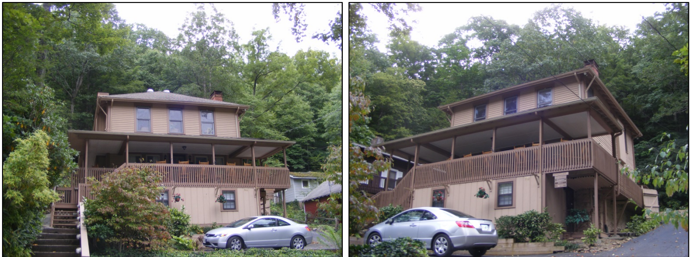
Figure 13. BN 5964: 302 Texas Road (Left: Façade; Right: Façade and West Elevation). TRC 2013.
