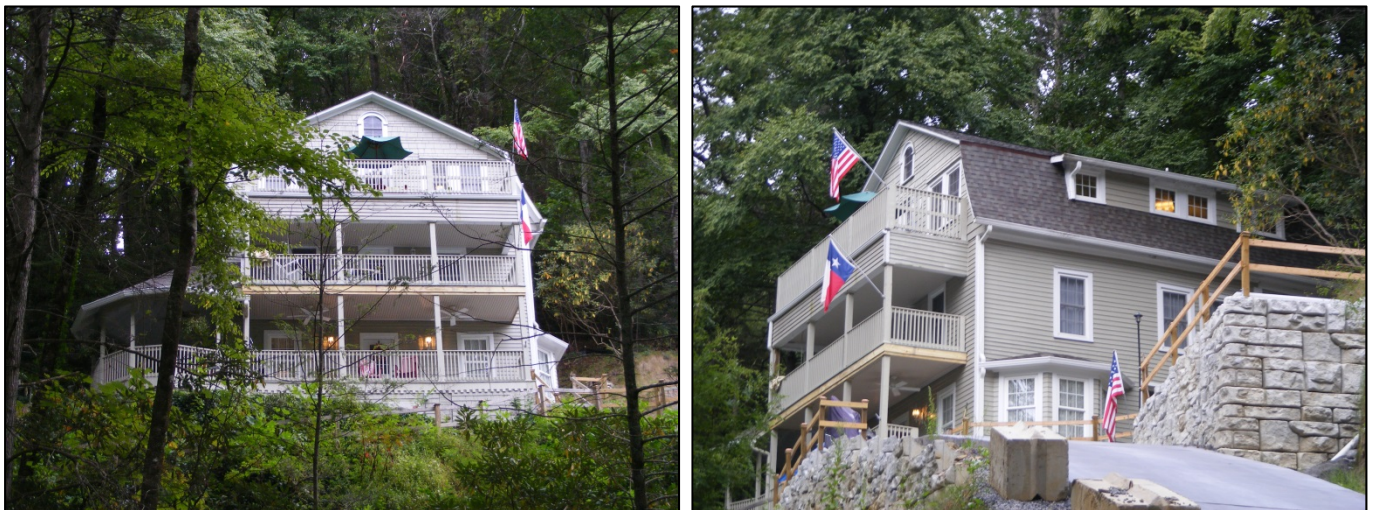
Figure 8. BN 5959: 238 Texas Road (Left: Façade; Right: Façade and West Elevation). TRC 2013.
