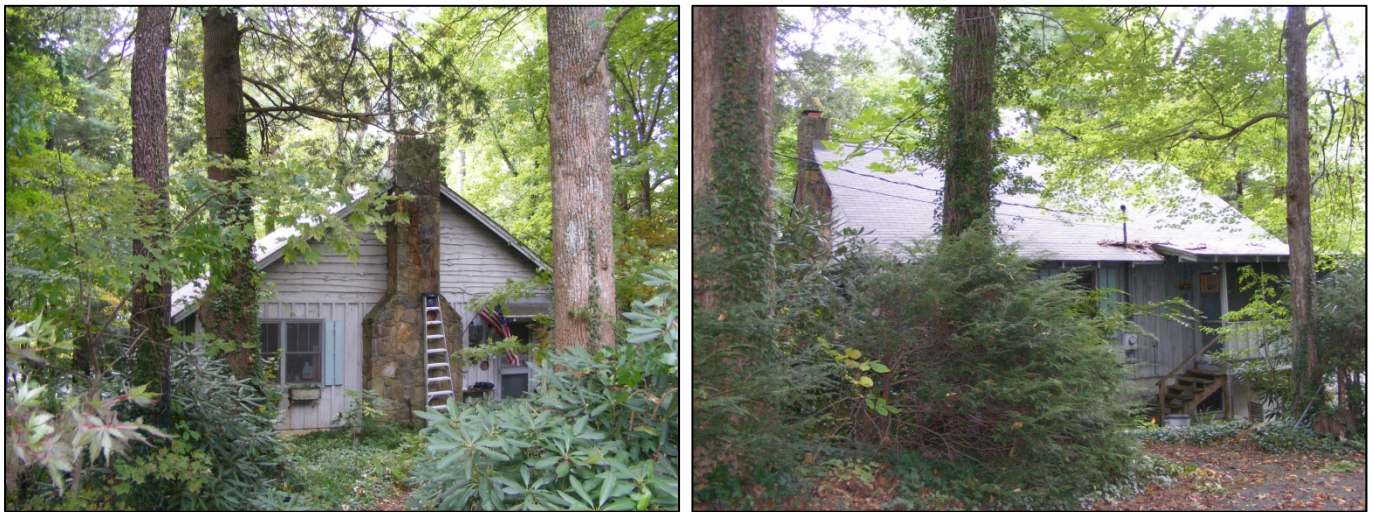
Figure 24. BN 5975: 220 Assembly Drive (Left: Façade; Right: West Elevation). TRC 2013.
