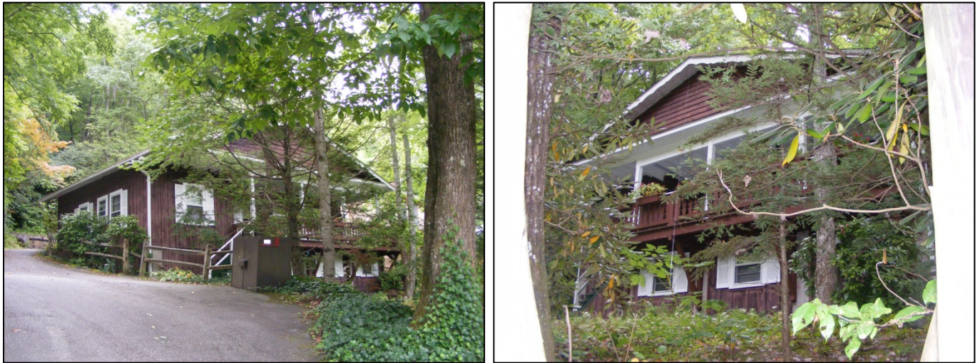
Figure 14. BN 5965: 304 Texas Road (Left: Façade and East Elevation; Right: Façade). TRC 2013.
