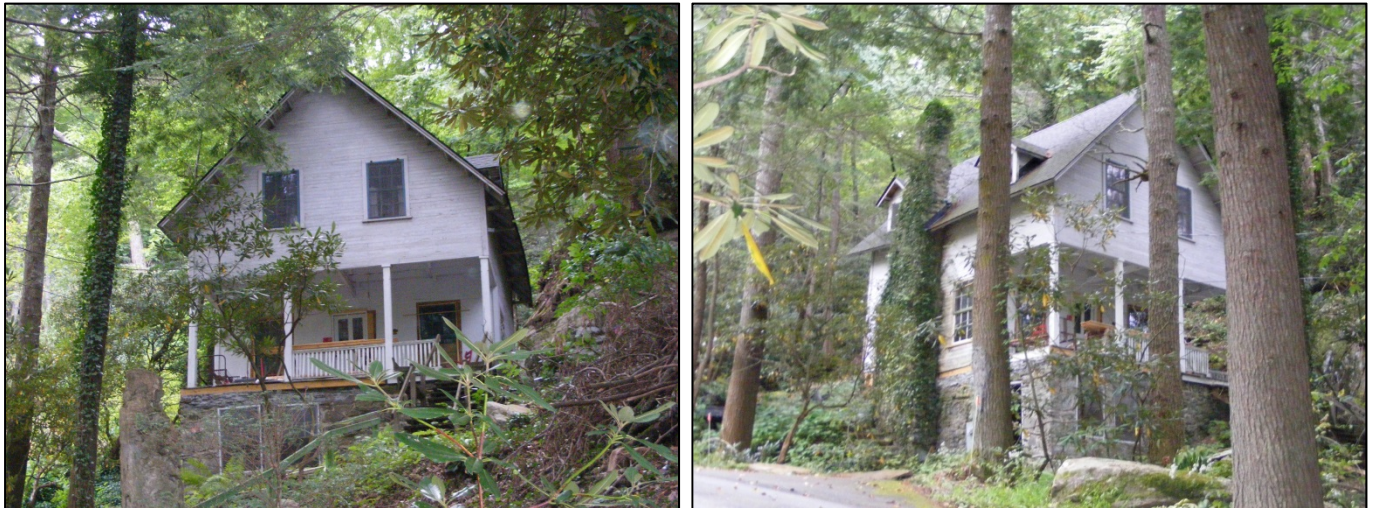
Figure 9. BN 5960: 242 Texas Road. (Left: Façade, Right: Façade and East Elevation). TRC 2013.
