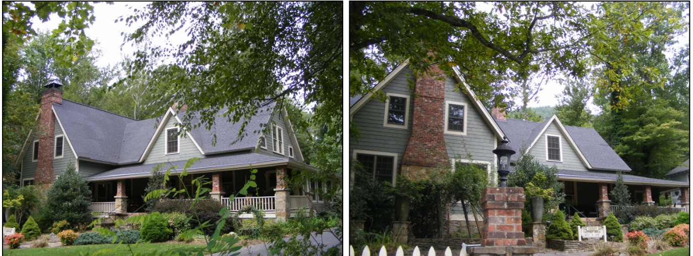
Figure 29. BN 5980: 237 Assembly Drive (Left: Façade and East Elevation; Right: Façade). TRC 2013.
