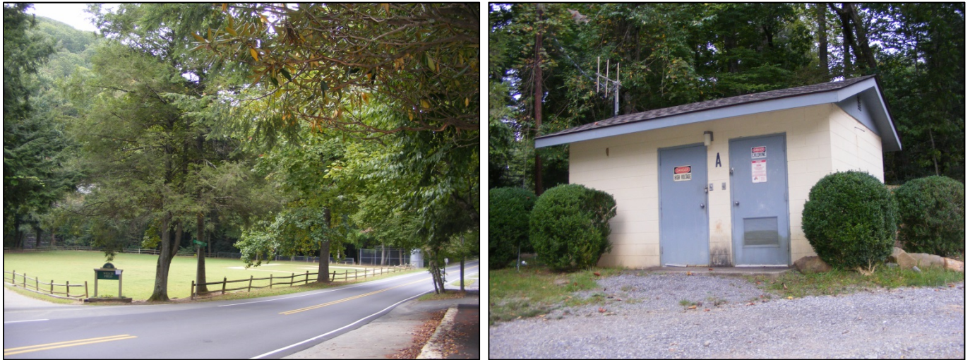
Figure 33. BN 5984: Welch Park (Left: Baseball Field and Path; Right: Well Building). TRC 2013.
