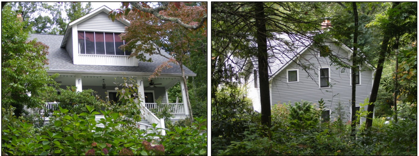
Figure 22. BN 5973: 218 Alabama Terrace (Left: Façade; Right: East and Rear Elevations). TRC 2013.
