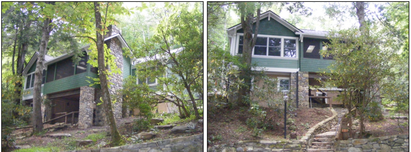
Figure 10. BN 5961: 246 Texas Road (Left: Façade and West Elevation; Right: Façade). TRC 2013
