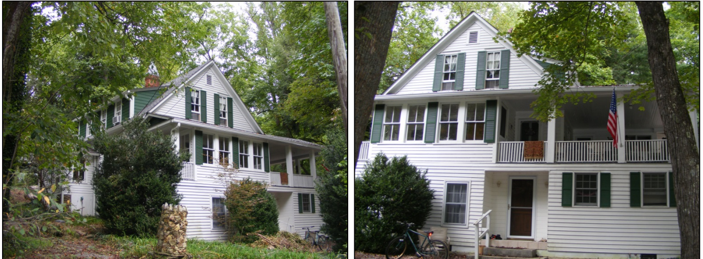
Figure 31. BN 5982: 231 Assembly Drive (Left: Façade and West Elevation; Right: Façade). TRC 2013.
