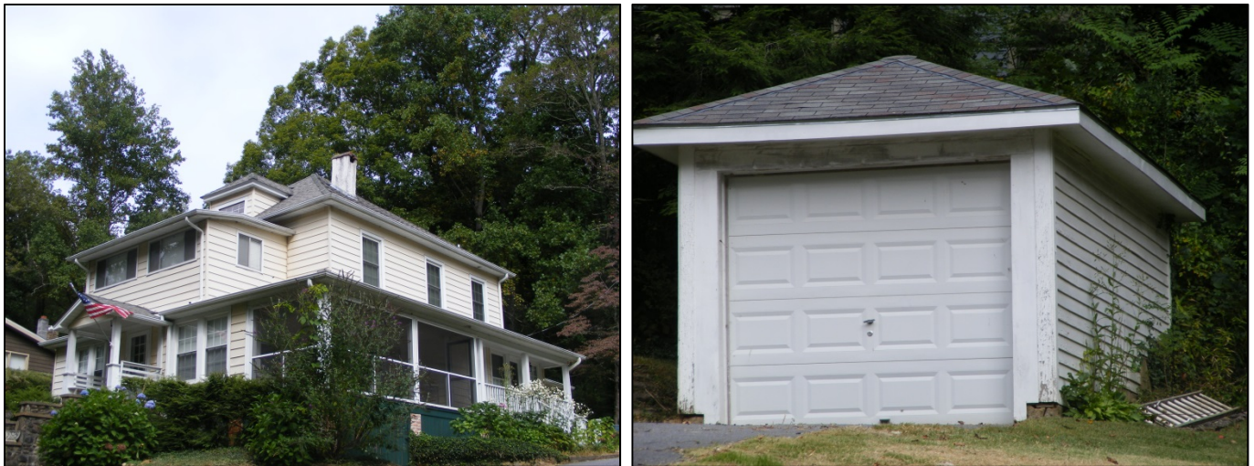
Figure 26. BN 5977: 223 Tennessee Road (Left: Façade and East Elevation; Right: Garage). TRC 2013.
