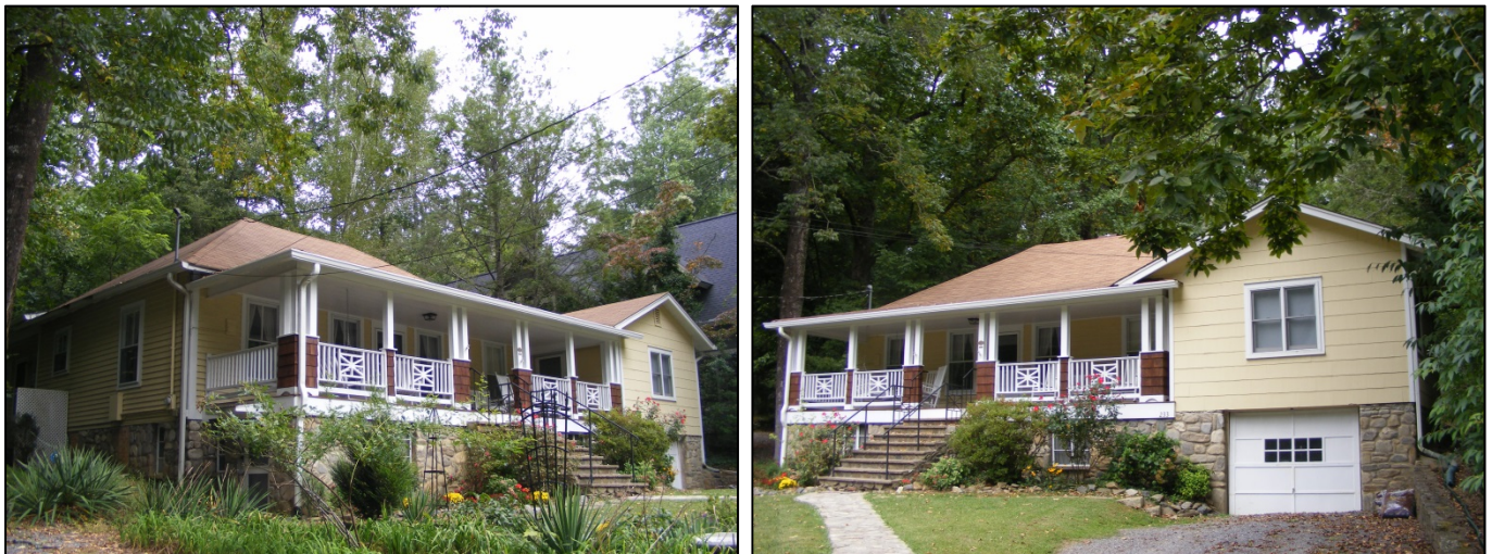
Figure 30. BN 5981: 233 Assembly Drive (Left: Façade and West Elevation; Right: Façade). TRC 2013.
