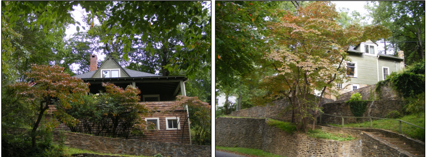
Figure 21. BN 5972: 222 Alabama Terrace (Left: Façade; Right: South Elevation and Stone Retaining Wall). TRC 2013.
