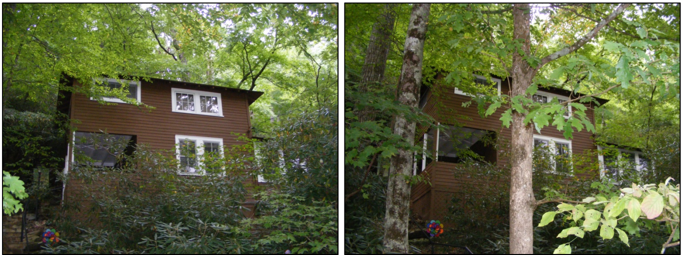
Figure 16. BN 5967: 312 Texas Road (Left: Façade; Right: Façade and East Elevation). TRC 2013.
